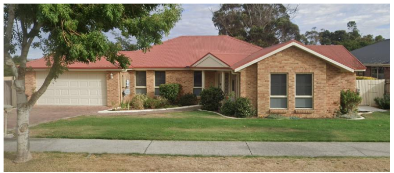
Figure 02 Solid pane, awning window (25 Cambock Lane West)
