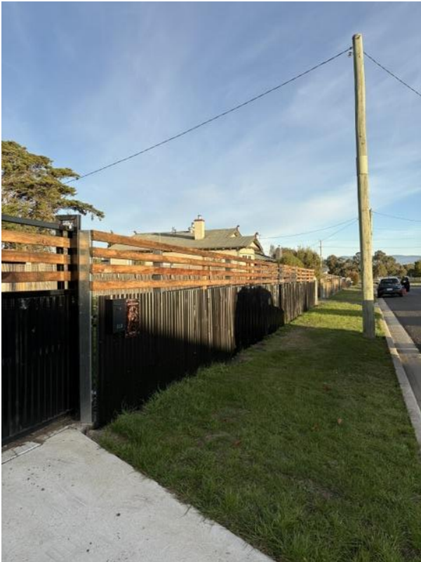
FINISHED FENCE AS IT CURRENTLY STANDS
