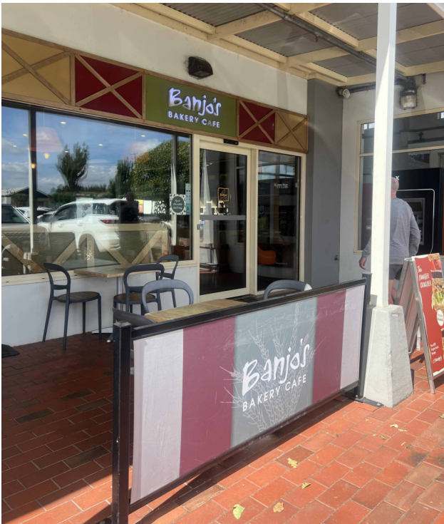
EXISTING STORE FRONT VIEW
