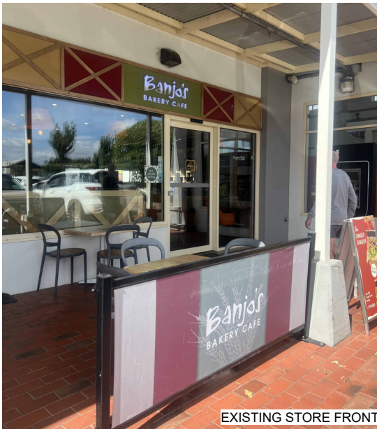
EXISTING STORE FRONT
