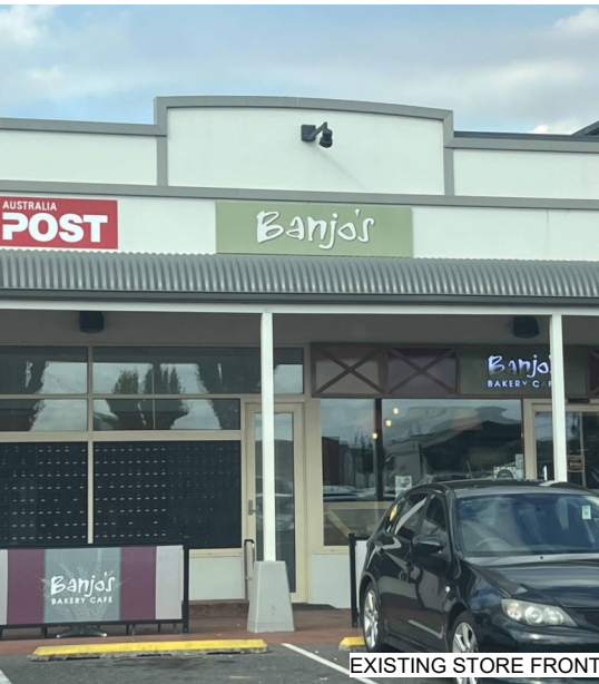
EXISTING STORE FRONT
