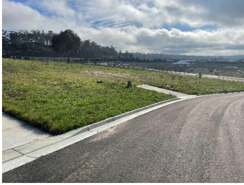
Figure 1. Lot 30 (subject site) crossover on the left, and the crossover of the adjoining property Lot 31 on the right.
