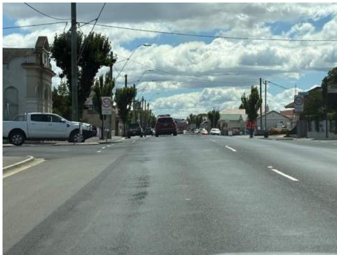
Figure 8 – Marlborough Street Southern approach
