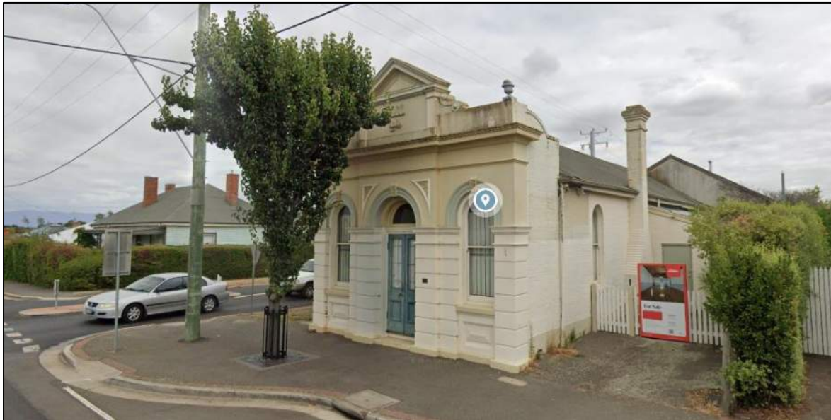
Figure 5: Marlborough St frontage showing original decorative parapet and hall entry (Source: Google Maps image February 2026)
