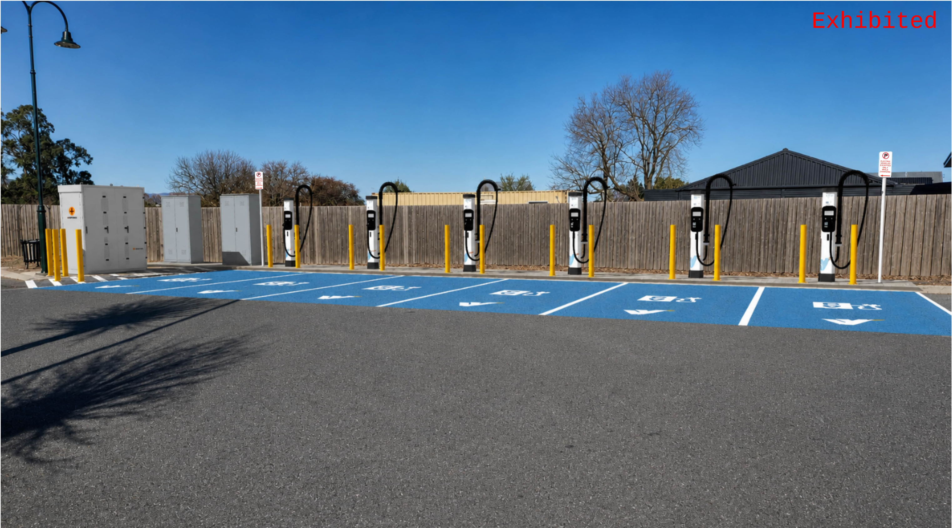
Existing 2 x Tritium chargers to be replaced by 6 x Kempower Single cable Satellite Chargers and 6 Vehicle Charging Bays
