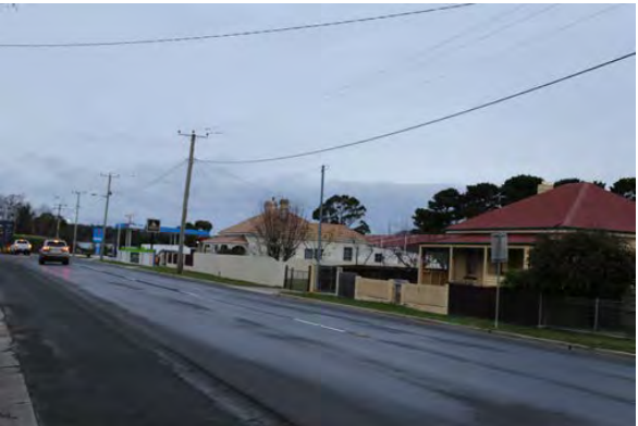
View looking south east along Main Road
