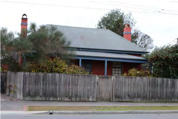
Residential dwelling within retail zone (Main Road)
