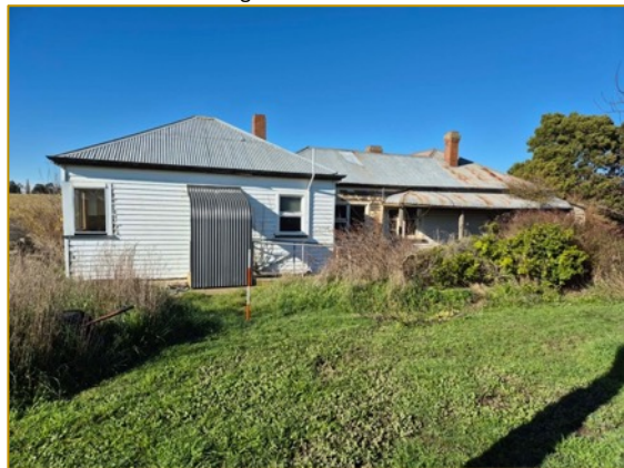
12. Rear, northern section of the house showing later extension.
