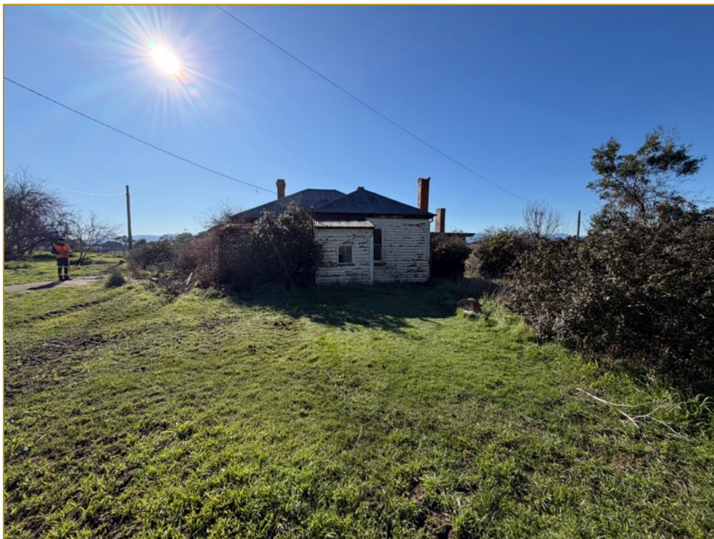
Figure 16: c1922 house looking east. Photograph by Darren Watton 11 th August 2026.
