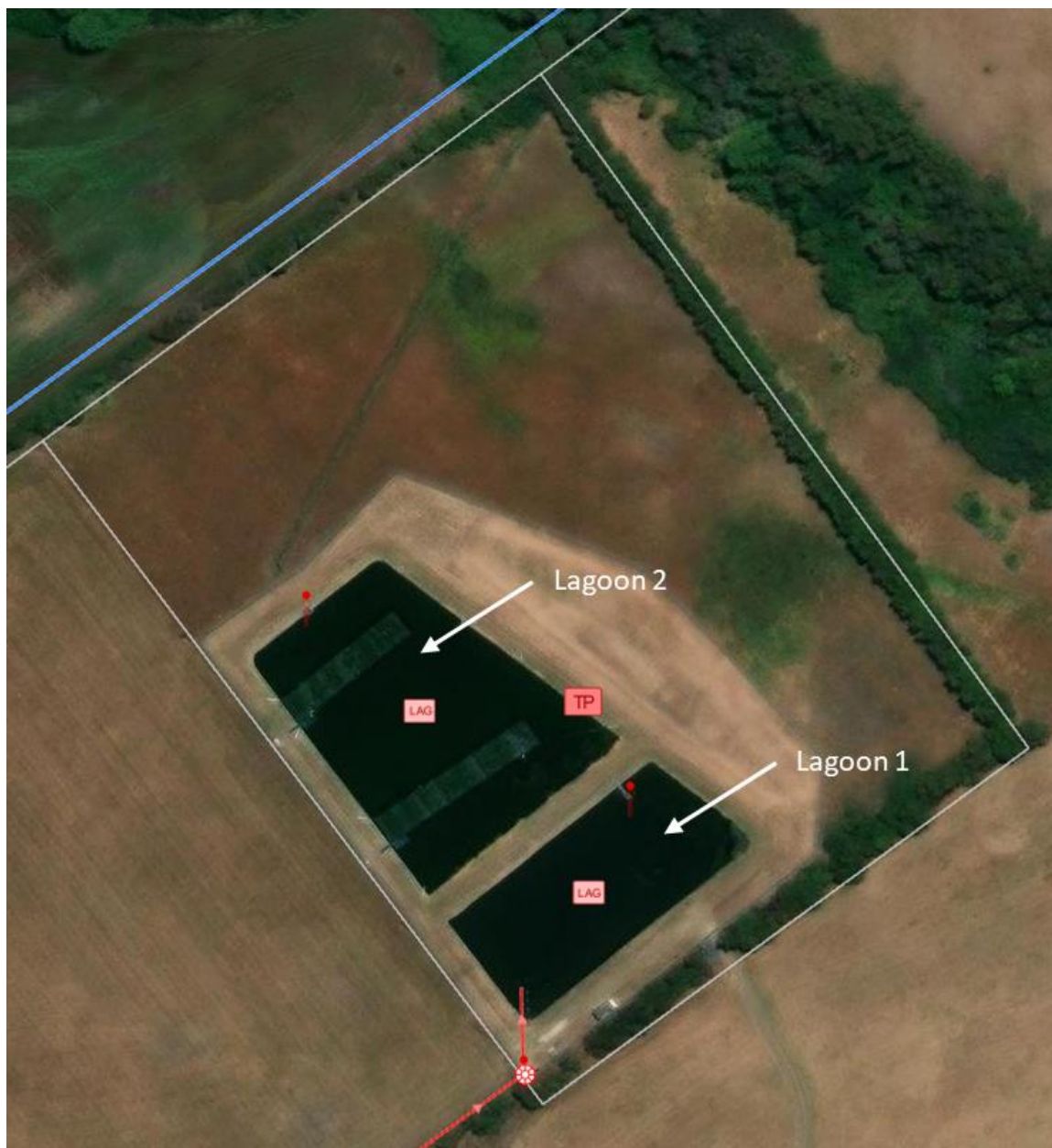
Figure 1. An aerial view of Western Junction STP showing the two treatment lagoons.
