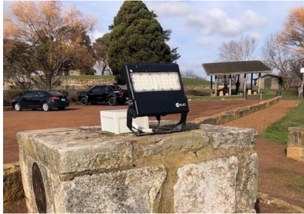
Ross Bridge flood light
