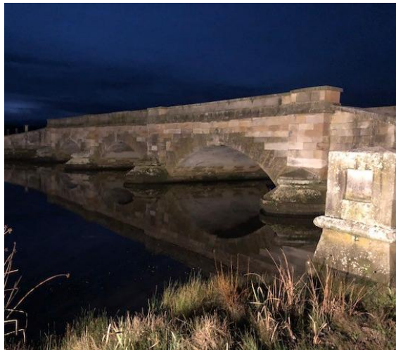
Flood lighting at the Ross Bridge
