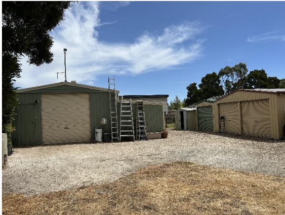
Figure 4 Existing outbuildings at rear of site.
