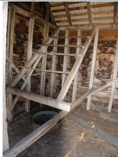
Interior of poultry shed (Space G25)
