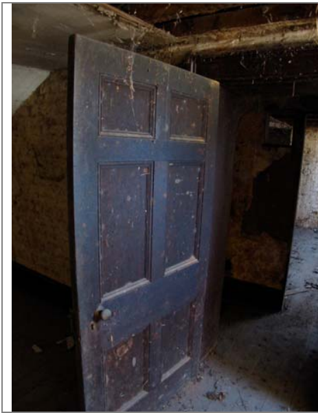
Door ? in attic
