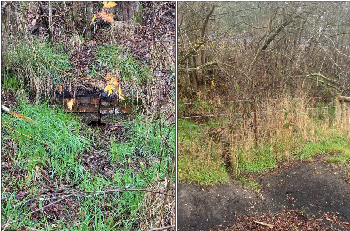
Figure 5. Photos of the TasRail culvert from site.
