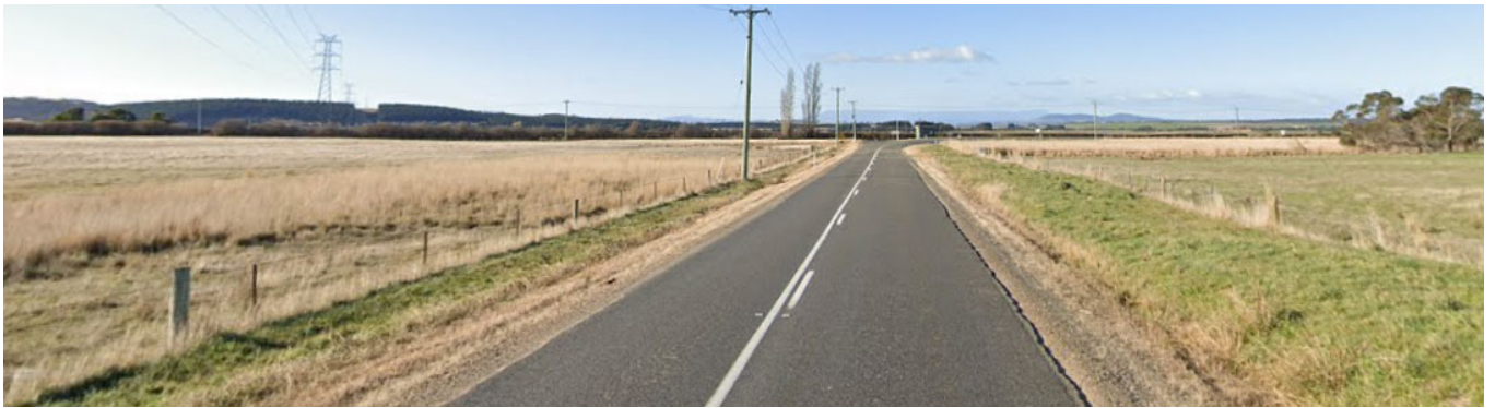
Figure 3 Poatina Road looking east, subject site on the left
