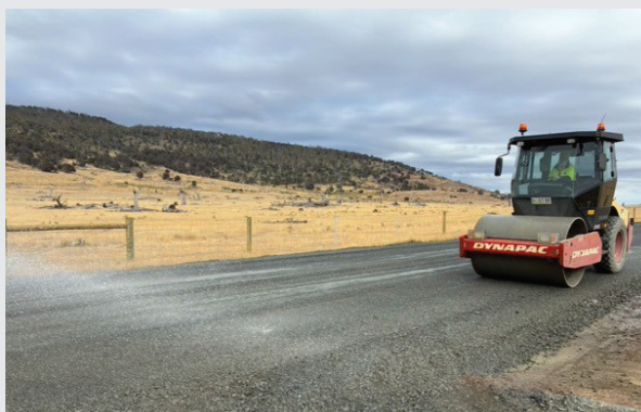
Construction crews undertake reconstruction and sealing works on Ashby Road, delivering improved road safety, reduced maintenance requirements and enhanced access for the local community.
