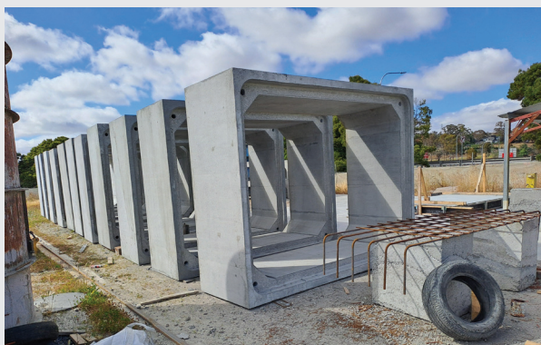
New culvert components ready for installation as part of Council's investment in maintaining and upgrading critical infrastructure across the municipality.
