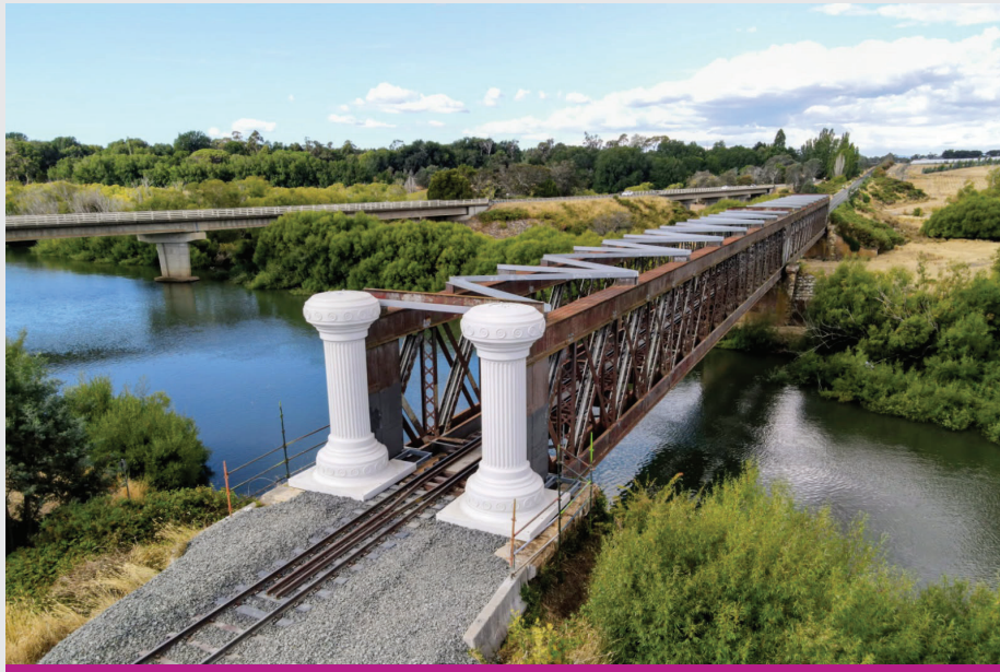
Longford Rail Bridge back to its beautiful glory with the newly installed columns. Photo by Fred Talavera.
