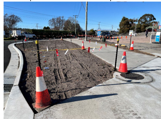
Perth Main Street foot path improvements.
