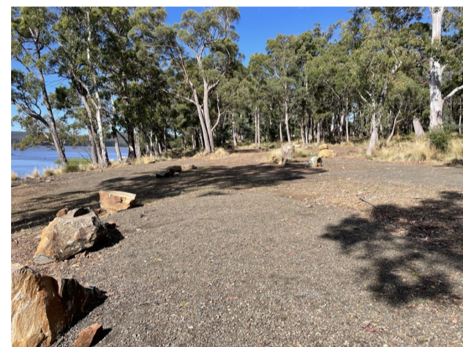
New compacted soil/gravel and rock placement.
