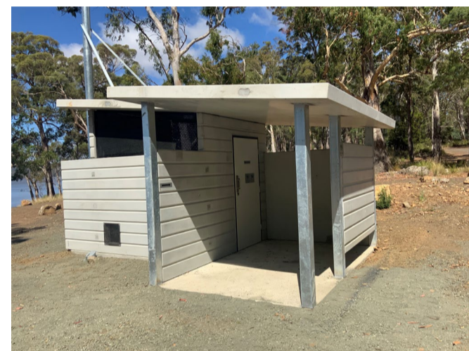
New pump out toilet facility.
