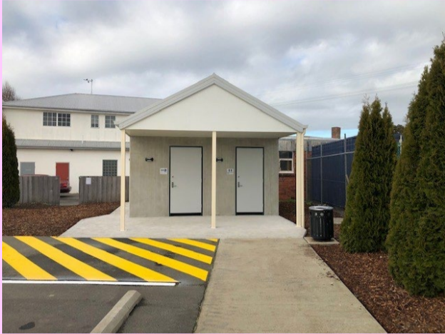
The rebuild of the public toilets in Talisker Street in Perth (behind the IGA)
