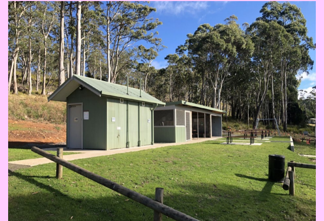
Upgrades to the toilet/shower facility at Lake Leake campground.
