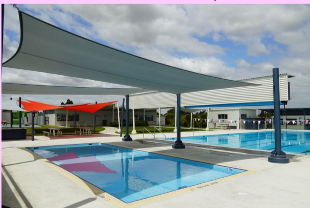
Cressy Memorial Swimming Pool upgrades.
