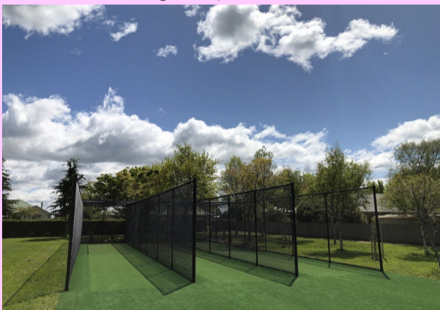
Morven Park Cricket nets were replaced.
