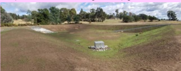
Gatty Street Detention Basin in Western Junction was designed to deal with the run-off from a 1 in 100-year storm event.
