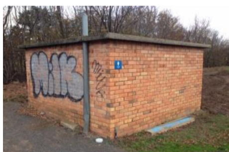
Former old toilet/shower block
