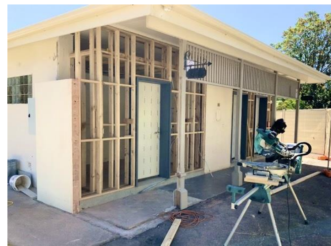
New façade taking shape on the amenities.
