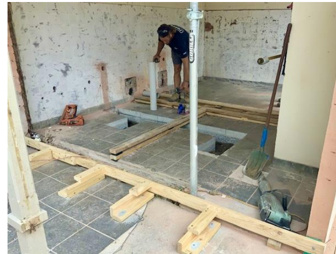
Work in progress on the plumbing and sewerage.
