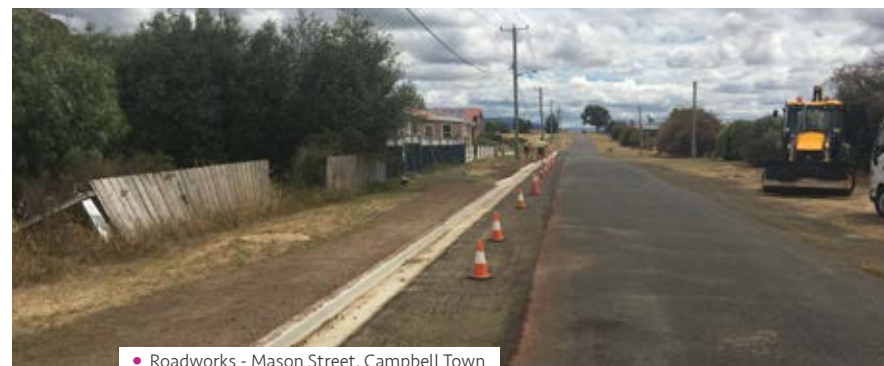
• Roadworks - Mason Street, Campbell Town
