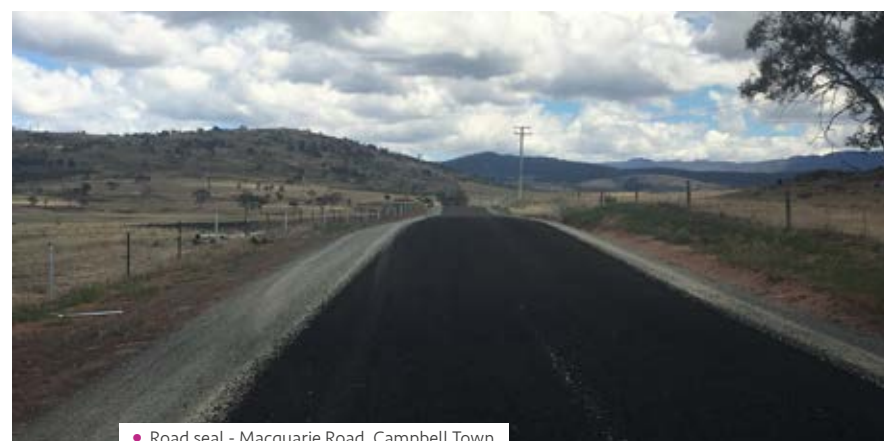
• Road seal - Macquarie Road, Campbell Town
