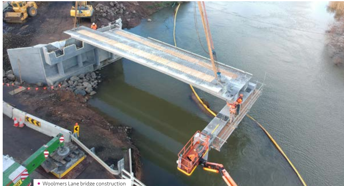
• Woolmers Lane bridge construction
