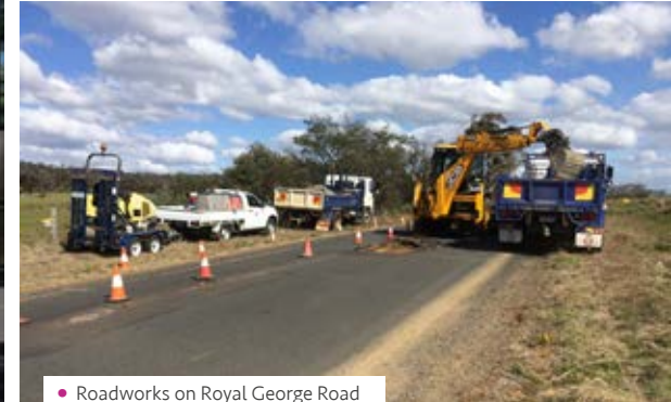
• Roadworks on Royal George Road
