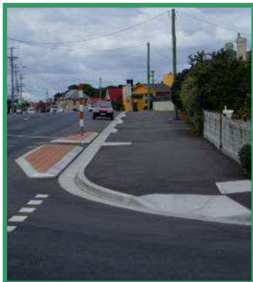
Upgrade of Main street, Perth
