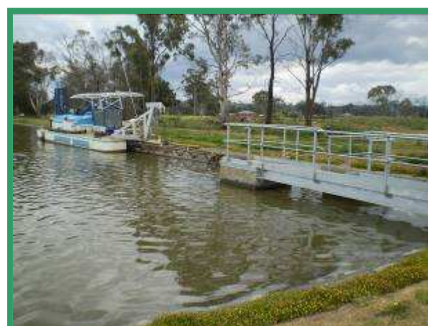
Longford Sewer Lagoon walkway improvements
