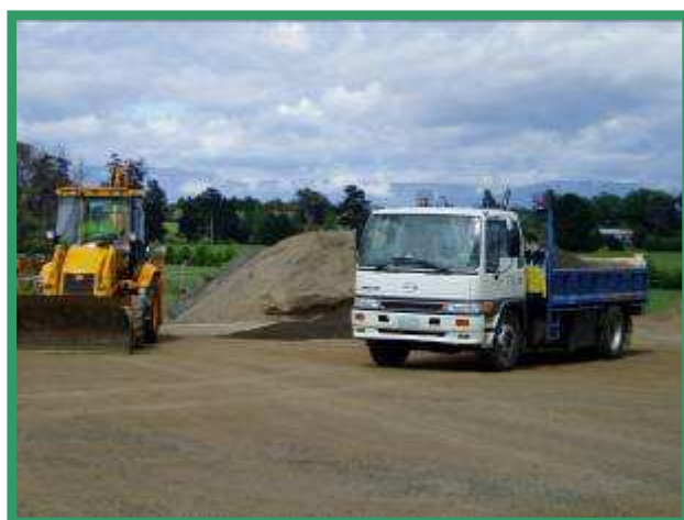
Storage of Materials at Hay Street Depot
