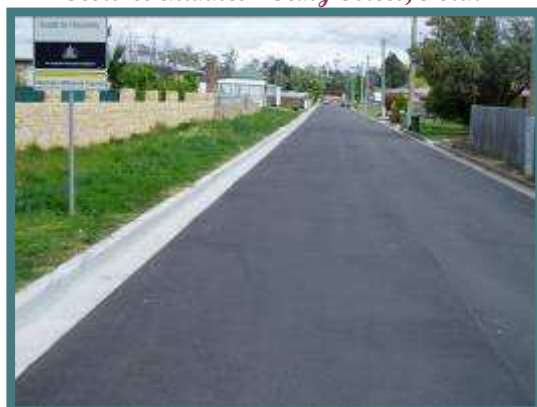
Kerb & channel - King Street, Perth
