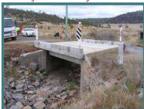
Bridge 5670 Deddington Road
