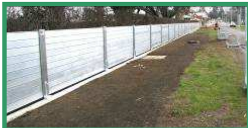
Erection of the temporary flood protection system
