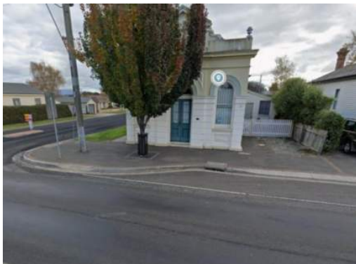
Figure 14 – Elevation view of driveway access to 38 Marlborough Street
