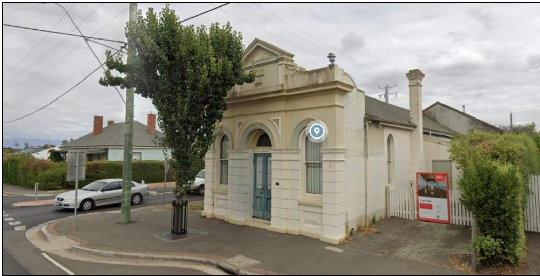
Figure 5: Marlborough St frontage showing original decorative parapet and hall entry (Source: Google Maps image February 2026)
