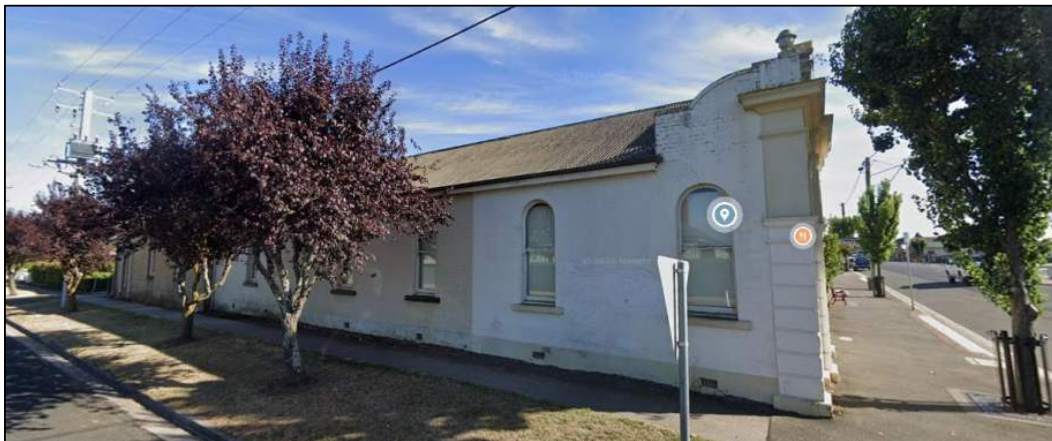
Figure 6: High St frontage showing original hall with feature windows and parapet façade (Source: Google Maps image February 2026)
