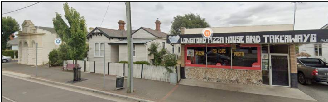
Figure 11: Properties situated to the north, including a dwelling house and food and drink outlet (Source: Google Maps image February 2026)
