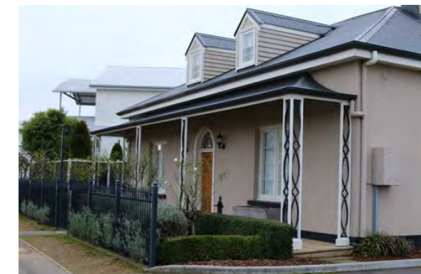
View of new retail conversion along Main Road
