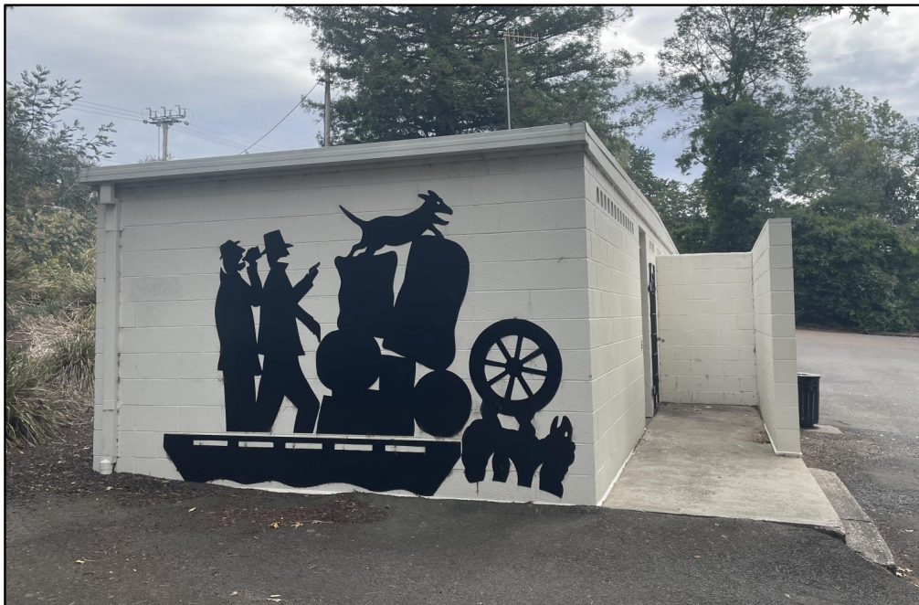
Toilet Facility Looking North
