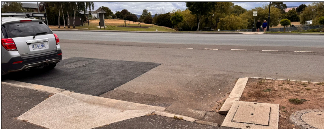
Figure 11 Pram ramps on northern side of Esplanade Intersection
