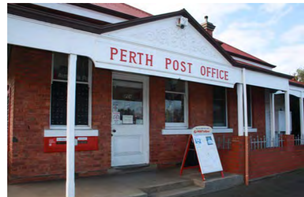
View of Perth Post Office (Main Road)
