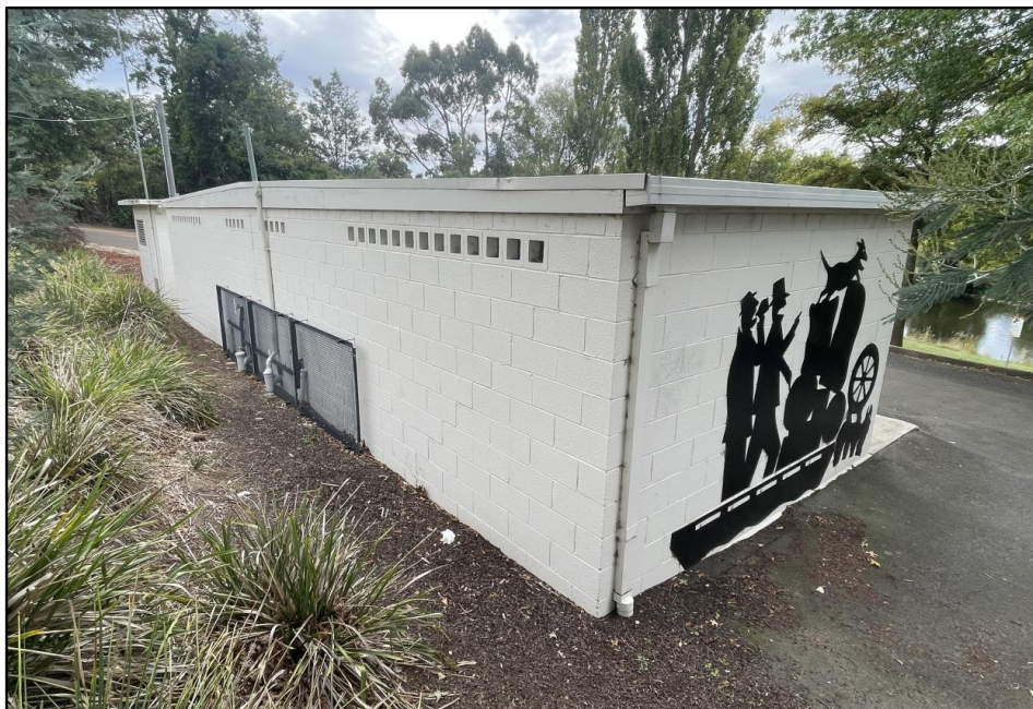
Toilet Facility Looking East
