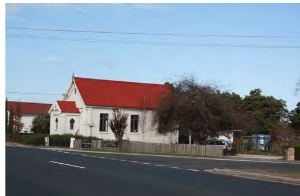
Adaptive re-use of former Church for Cafe (Main Road)
