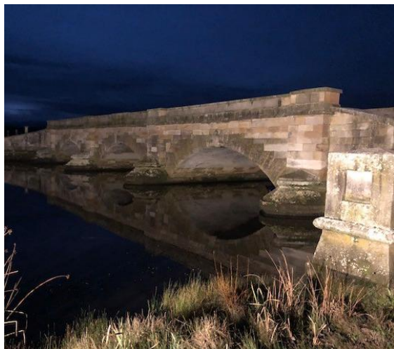
Flood lighting at the Ross Bridge
