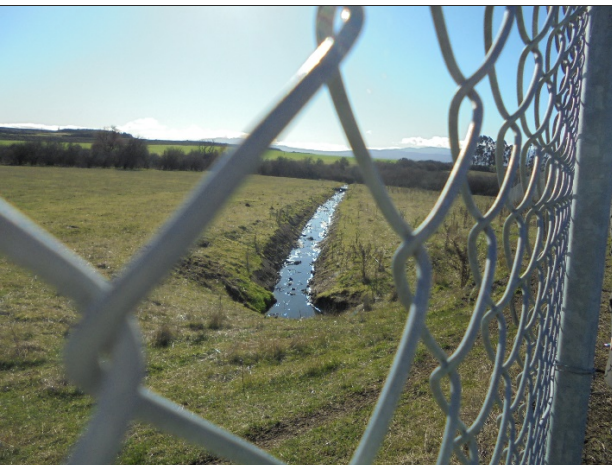
^open drain after leaving the lagoon system, draining to Briarly Creek
