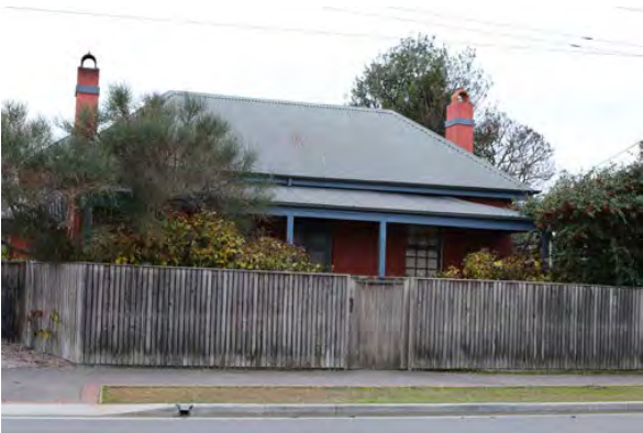
Residential dwelling within retail zone (Main Road)
