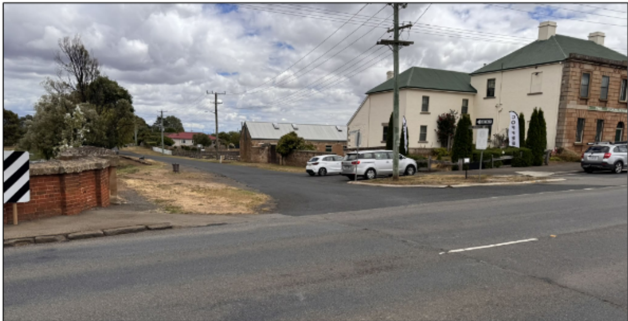
^Photographs of subject site
