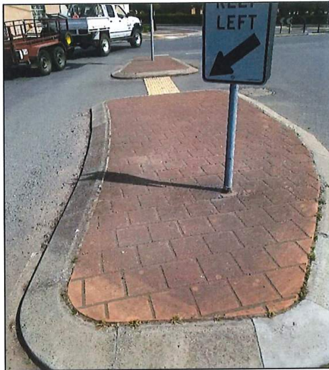
Photograph 3. Traffic island on the centreline of Wellington Street south
