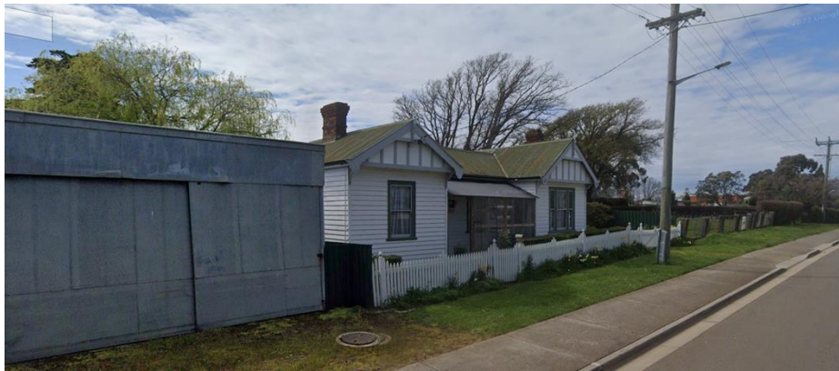
Image 2 Outbuilding of #23 Charles Street visible (left) with #8 Saundridge and currently vacant subject site to the right. Source Google Streetview.
