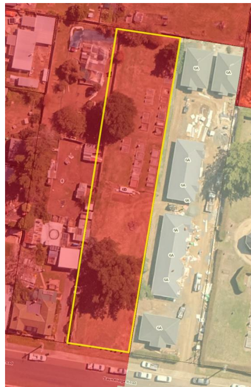
Photographs of subject site
