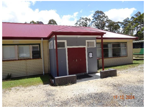
Photographs of subject site
