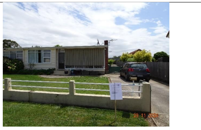
Photographs of subject site
