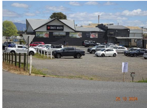
Photographs of subject site
