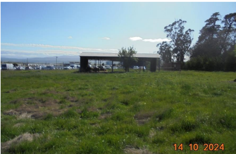
Figure 5 - shed to be demolished on subject site
