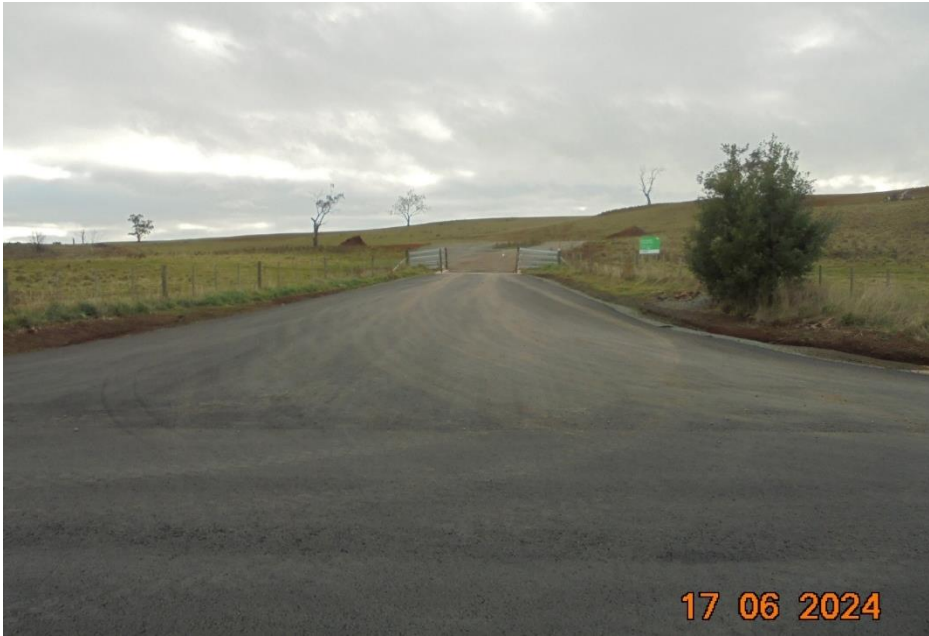
^ Entrance to Subject Site from Macquarie Road
