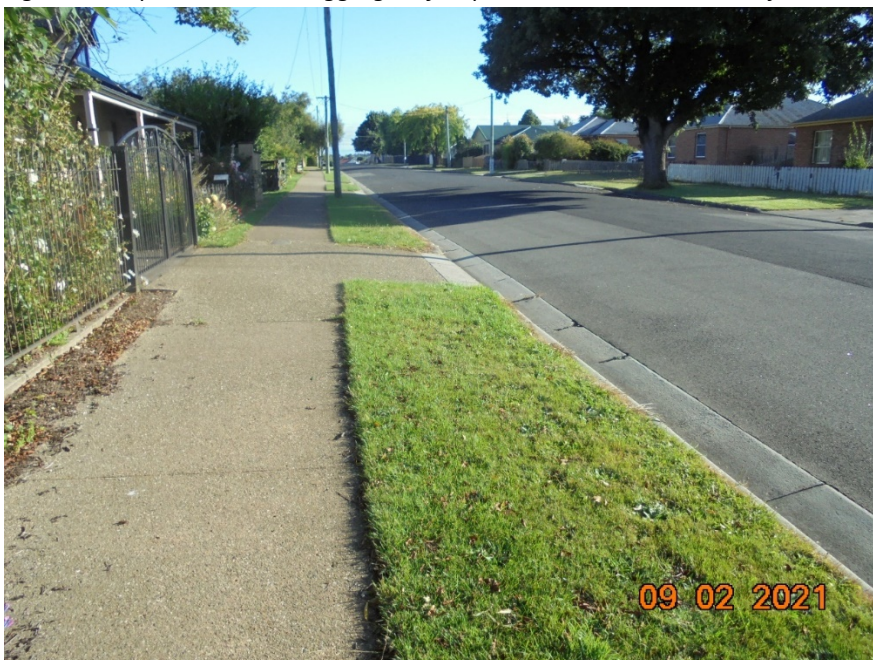
Figure 8 – exposed concrete aggregate footpath in Scone Street and adjacent crossover
