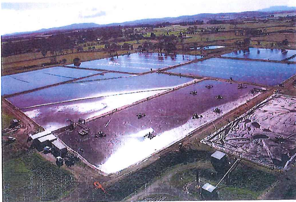
Figure 3 - Aerial View of Longford STP
