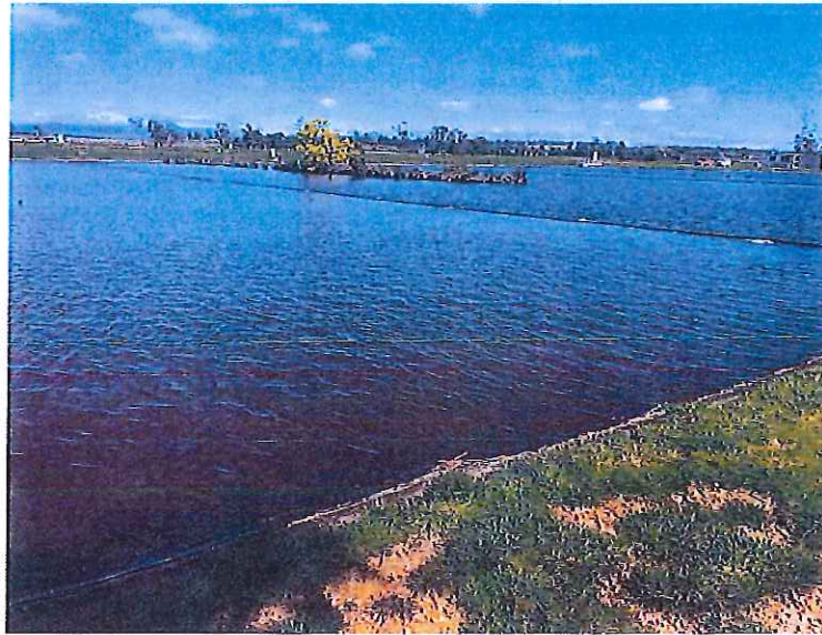
A settling pond associated with the treatment of sewage.
