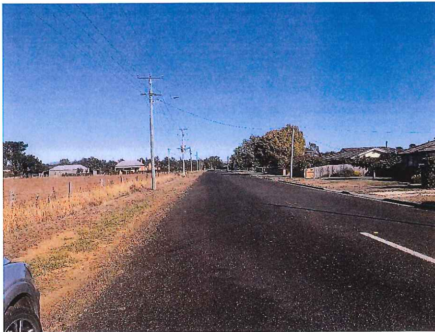
Figure 7 – Bulwer St looking west
