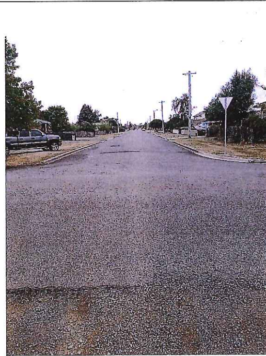
Figure 6 - looking north along Burghley Street
