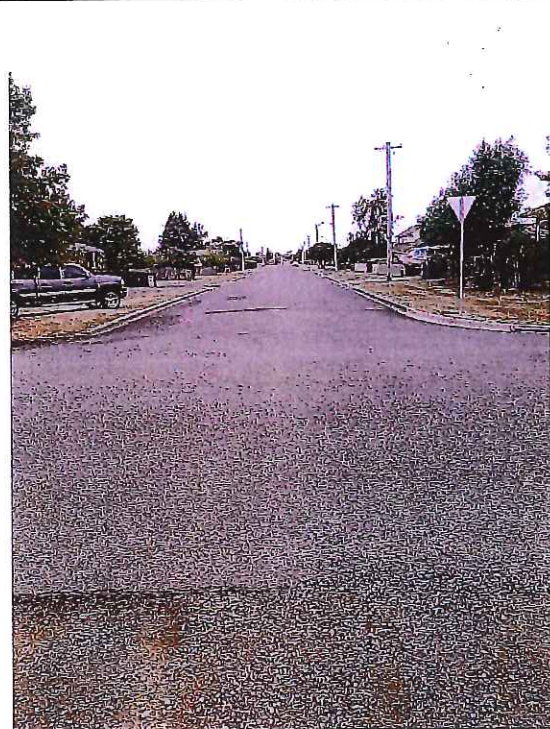
Figure 6 - looking north along Burghley Street
