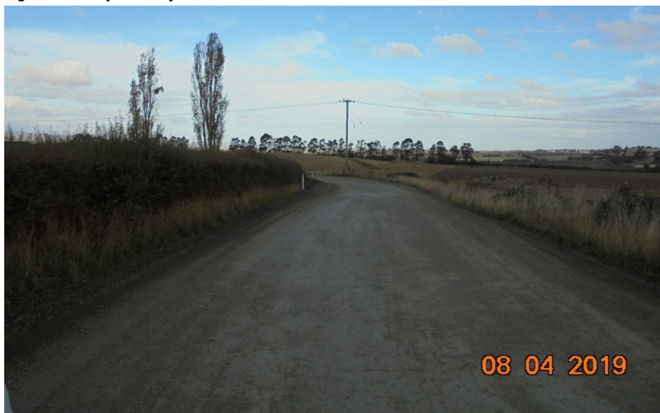
Figure 1 - Subject site from internal access road
