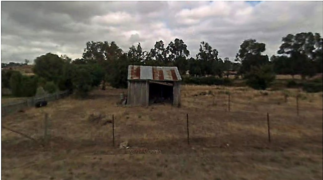
Shed to be demolished
