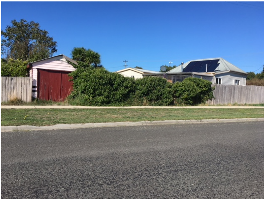
^ 45 Clarence Street, constructed on the northern boundary
