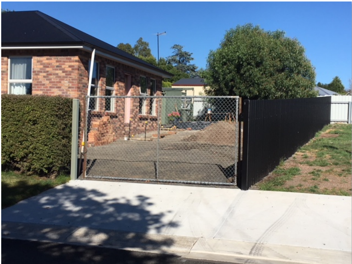
^ Boundary between 12 and 12A William Street, noting physical separation, driveway location, window sill height and boundary fencing and existing landscaping
