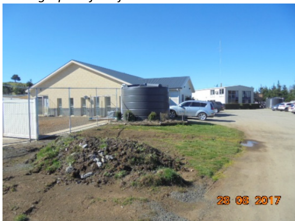
Photographs of subject site
