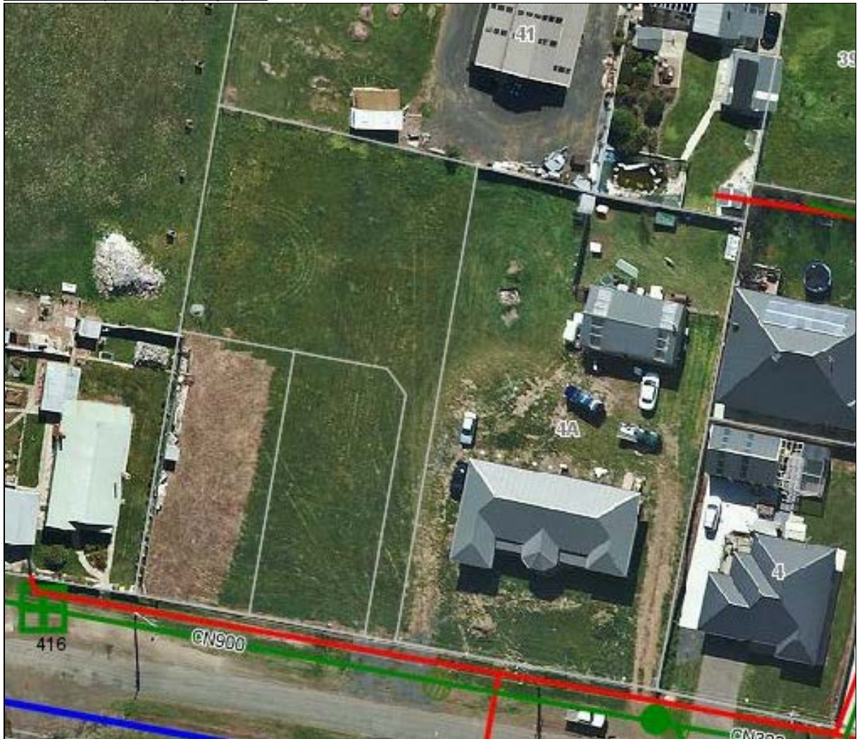
Photographs of subject site
