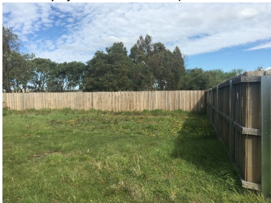
Looking south from end of access (along boundary of 5 Rose Gold Court)
