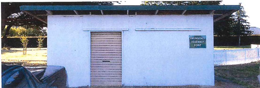
Figure 23 – Existing old change room.
