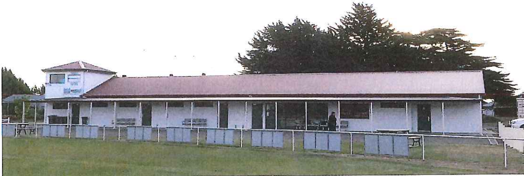
Figure 22 – Existing clubhouse and change rooms.
