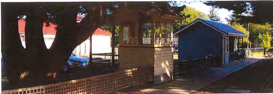
Figure 26 – Existing miniature railway station and control building.
