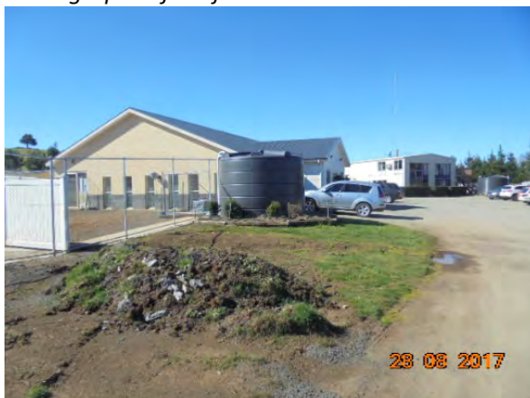
Photographs of subject site
