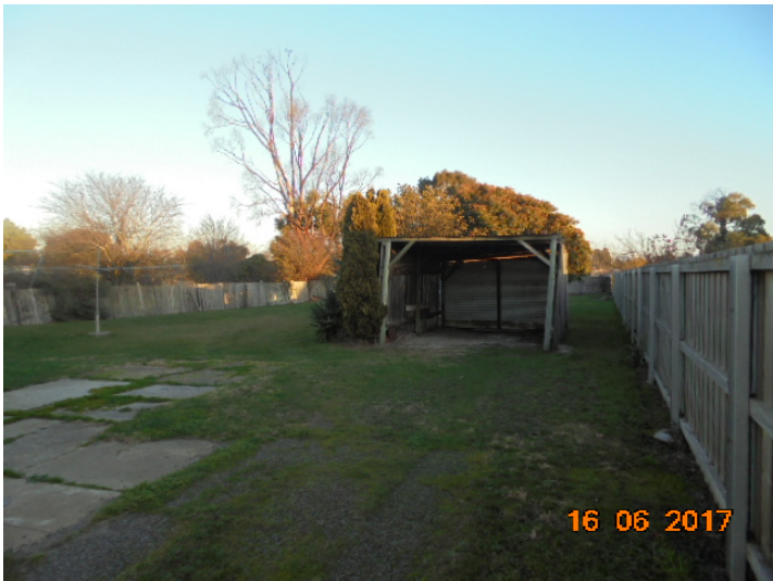
^Existing carport to be demolished
