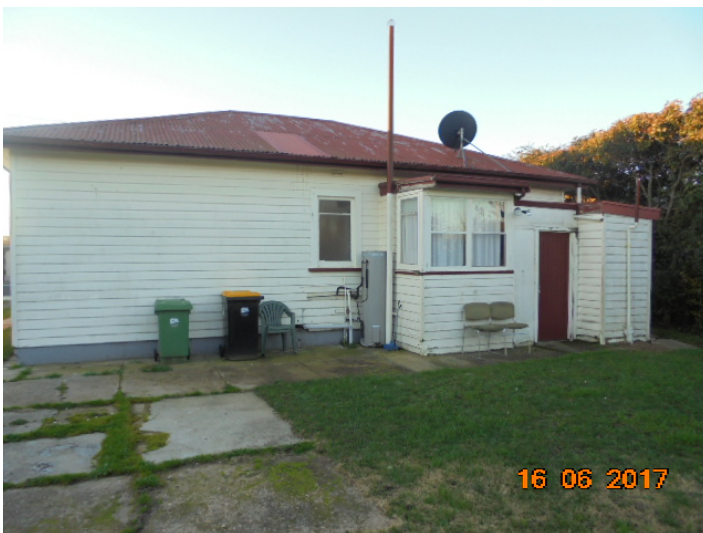
^ The rear of the existing dwelling (unit one).
